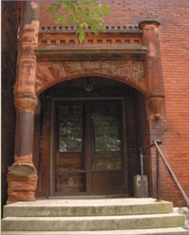
An animated doorway, like this one in Old Louisville, is a characteristic which adds to the charm of many historic neighborhoods in Louisville.
