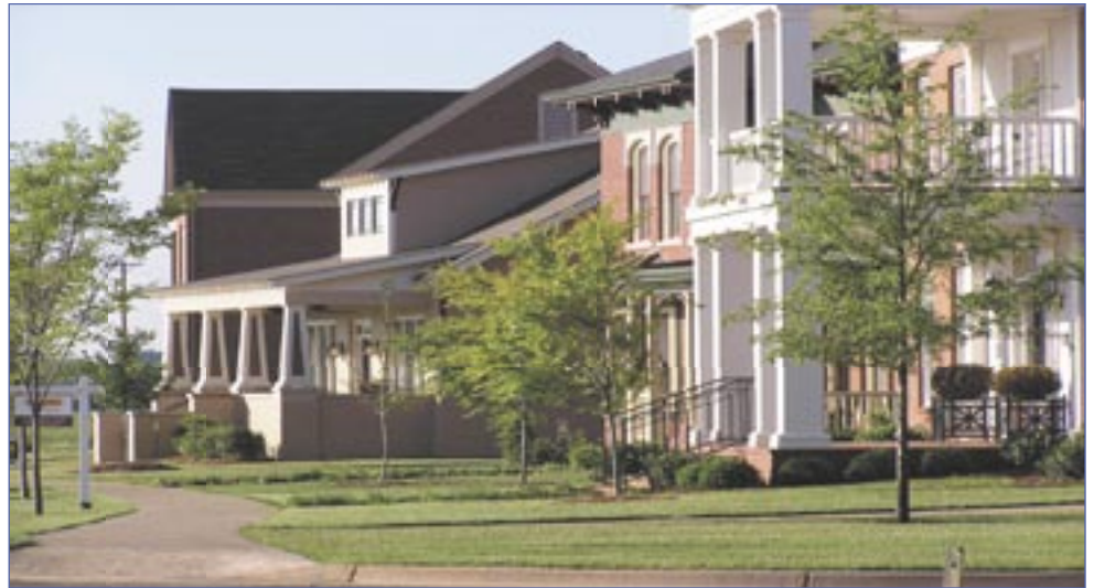
New construction in Norton Commons represents Cornerstone 2020's emphasis on architectural compatibility with surrounding structures.
